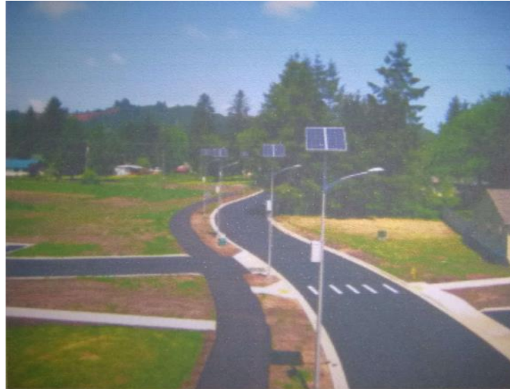
Figure 3: Solar Powered street light
